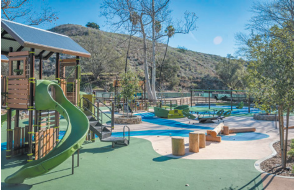
Construction for the play area began in early May 2021.
